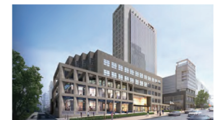
S-TOWER Remodeling (1st and 2nd construction) Client : Global SAE-A Scope : C Location : Seoul, Korea Execution period : 2018. 10 ~ 2021. 04
